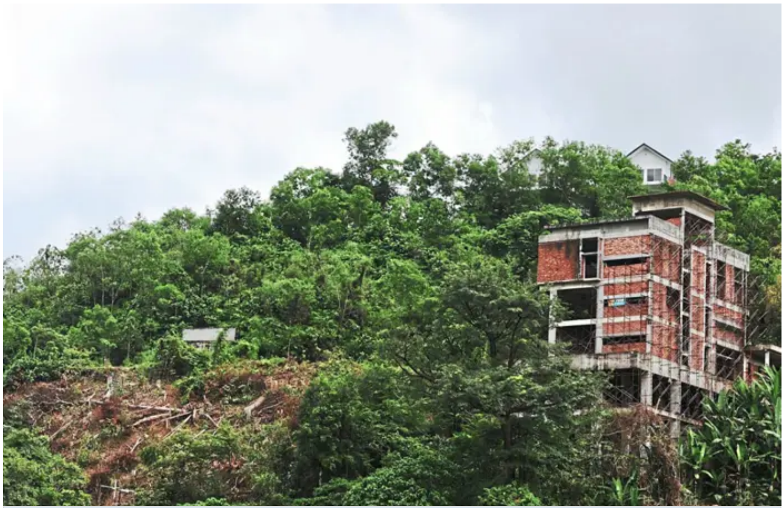
Hill slope development in places like Taman Melawati in Hulu Kelang is cause for concern among nearby residents. — AZMAN GHANI/The Star
