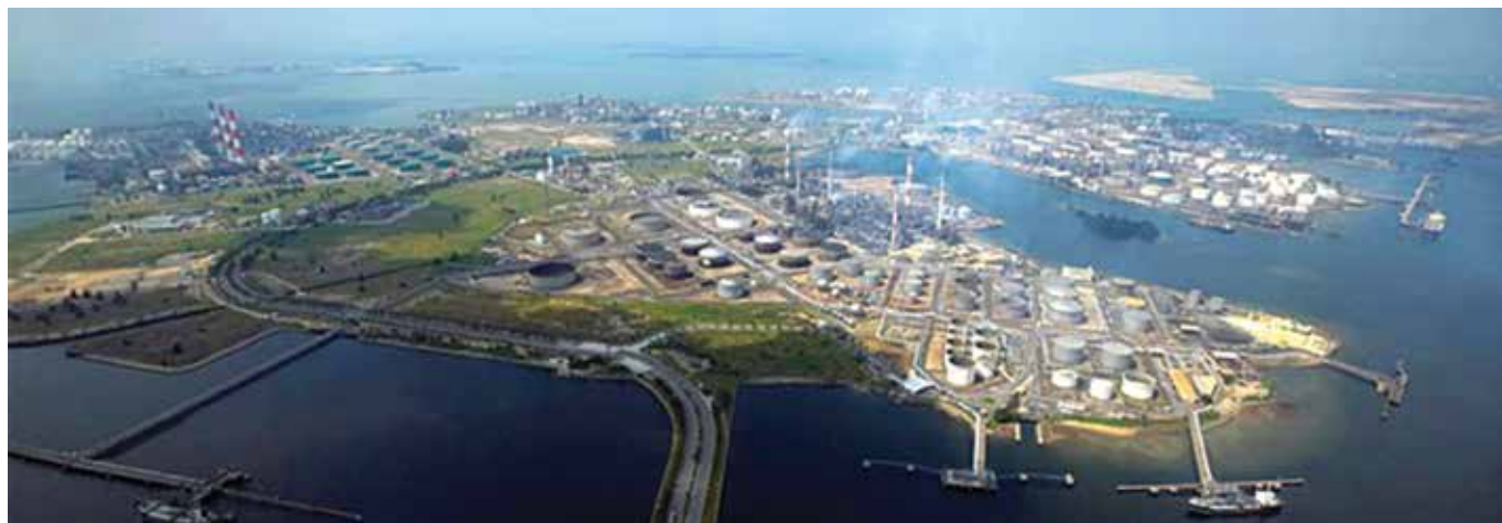
Jurong Island which houses top companies in Singapore's chemical industry will be the location for the fifth desalination plant
